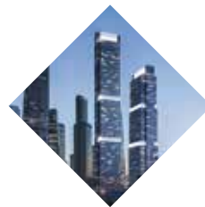
МФК Neva Towers
